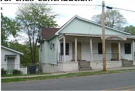
Future Home of the Christian Service "Ledbetter Heights" Learning Center
